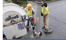
Sewer main cleaning is also done for CCTV inspection work. These inspections allow us to see the condition of our sewer mains and make necessary repairs or replacements.
